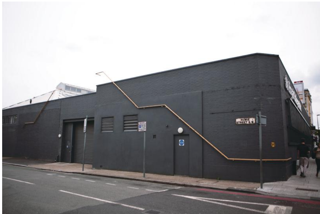
Distant Stairway 2011, Wooden handrail, brass, steel, 2780 × 150 × 690 cm
