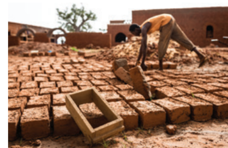
French National Commission for UNESCO: rammed-earth construction in Senegal with the not-for-profit association The Nubian Vault © The Nubian Vault/Régis Binard
